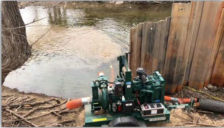
Construction Dewatering:
